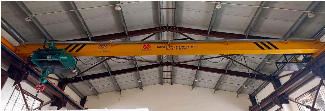
Some advanced laboratory facilities
