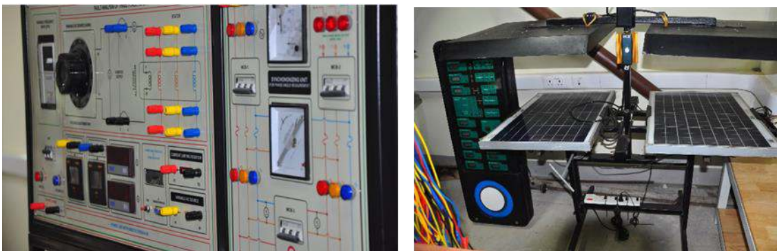
Power Systems Lab, Left: Alternator Fault Simulator With Grid Synchronization Facility, Right: Solar PhotoVoltaic Array Simulator
